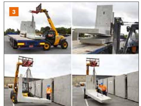
**1** The Forterra QuickLift system has been developed to ensure that no additional lifting equipment is needed other than conventional chains and hooks for the three lifting points. Unlike many other systems we have no hidden costs for expensive lifting gear.
