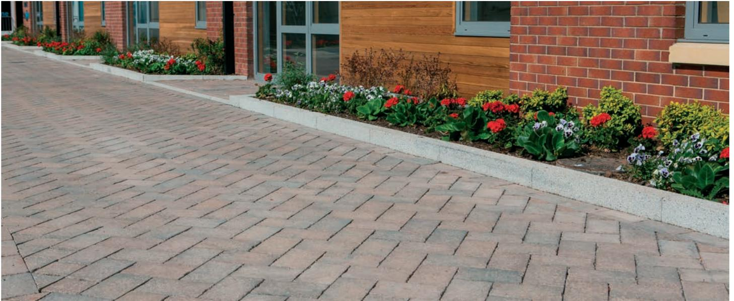
Installing a permeable paving sustainable urban drainage system (SUDS) eradicates surface pooling and puddles while allowing rainwater to be harvested and reused. Its use can reduce the risk of flooding and help control the amount of water that enters the drainage infrastructure.
