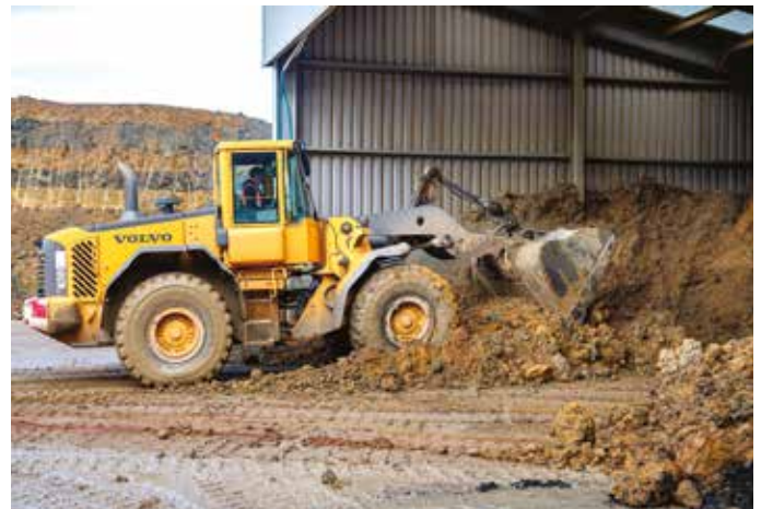
Extracted clay is stored in a stock pile
