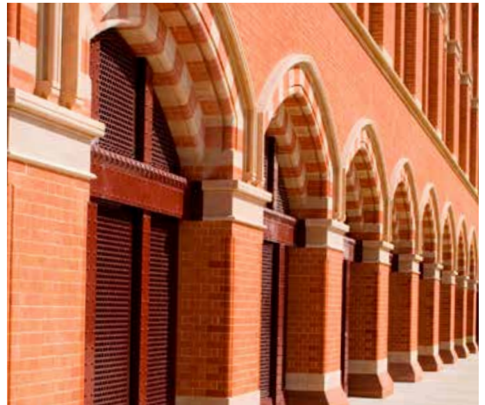
St Pancras Station Detail
